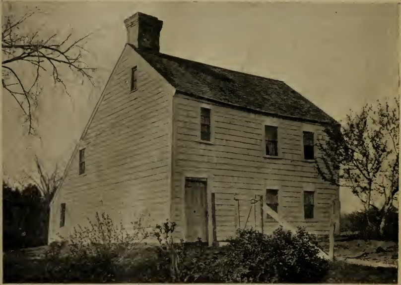
SAMUEL BOARDMAN HOUSE, ONE OF THE OLDEST IN ESSEX COUNTY, SITUATED OPPOSITE THE FORK OF THE WAKEFIELD AND MELROSE ROADS
